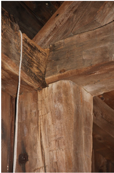
Top Left: example of English Tying Joint at 218 Dutton Hill Road; Top right: diagram of the joint from The English Barn in the New World/MAdisonbarns.wordpress.com
