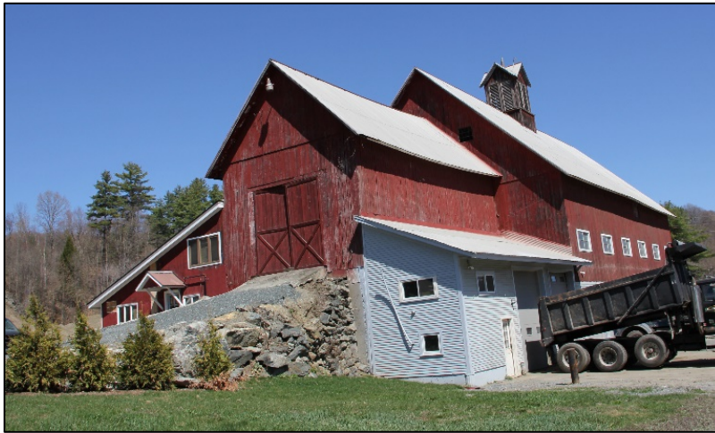
Top Left: High Drive bank barn at 287 River Road with stone abutment; Top Right: framing of the third level with upper loft platform.
