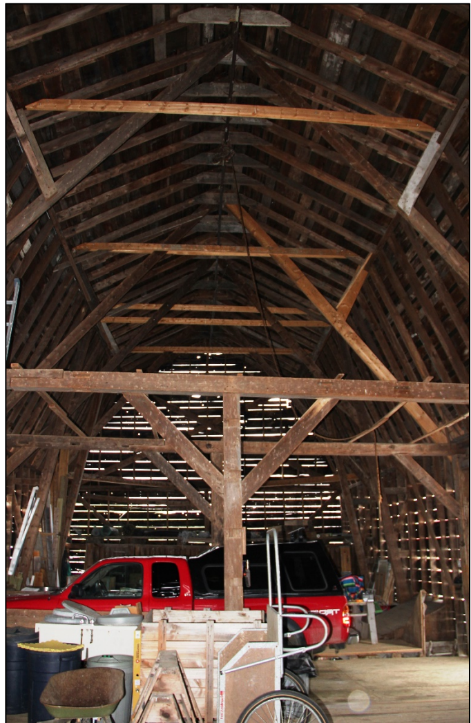
Left: 1910 plate from The Farmstead by I.P. Phillips, showing how to convert a gable to a gambrel; Top Right: 70 Cossingham barn with windowless upper levels and concrete basement stable; Bottom Right: interior of hay loft at 70 Cossingham with older timber frame below a more modern scissor truss-gambrel
