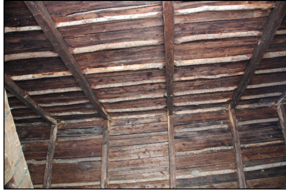
98 Campbell Flat Road: Left, scribe match marks on the frame; Right, principal rafters with common purlins pegged into them – an old style of roof framing uncommon in Vermont, but seen in Southern New England
