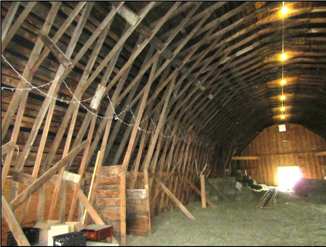
Top Left: ca. 1950 lister photo of the newly re-located Ground Level Stable barn at 752 Route 132 (Clark Farm) showing its original metal roof ventilators, stable windows, extended roof peak to protect the hayfork machinery; and its attached milk house; Top right: The ca. 1939 Thetford gambrel roofed barn of Roy Clark's brother; Bottom Left: The stick framing of the gambrel roof at 752 Route 132; Bottom Right: The original metal cow stanchions.
