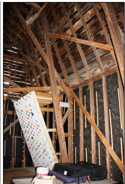
Bottom Left: Photos of erecting the scissors truss type of gambrel roof frame from the Jamesway Co. Catalog of 1918; Bottom Center: Scissors truss in gambrel roof of 5 Happy Hill; Bottom Right: scissors truss at 70 Cossingham gambrel roof
