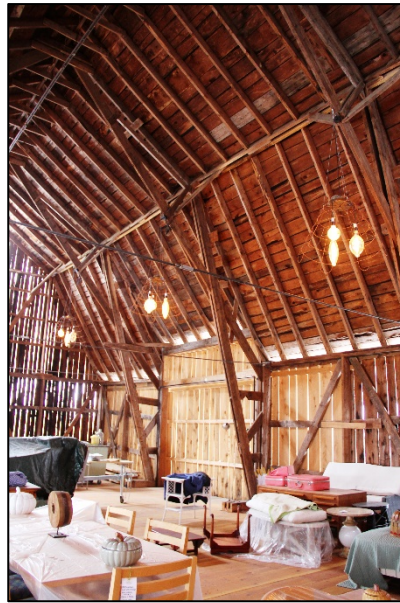
Bottom Left: Photos of erecting the scissors truss type of gambrel roof frame from the Jamesway Co. Catalog of 1918; Bottom Center: Scissors truss in gambrel roof of 5 Happy Hill; Bottom Right: scissors truss at 70 Cossingham gambrel roof
