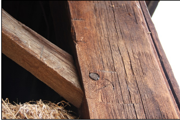
98 Campbell Flat Road: Left, scribe match marks on the frame; Right, principal rafters with common purlins pegged into them – an old style of roof framing uncommon in Vermont, but seen in Southern New England
