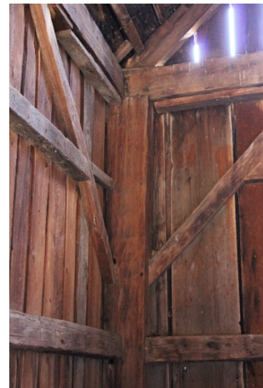
98 Campbell Flat Road: Bottom Left, entrance to former threshing floor; Bottom Right, gunstock post with English Typing Joint in 98 Campbell Flat Road
