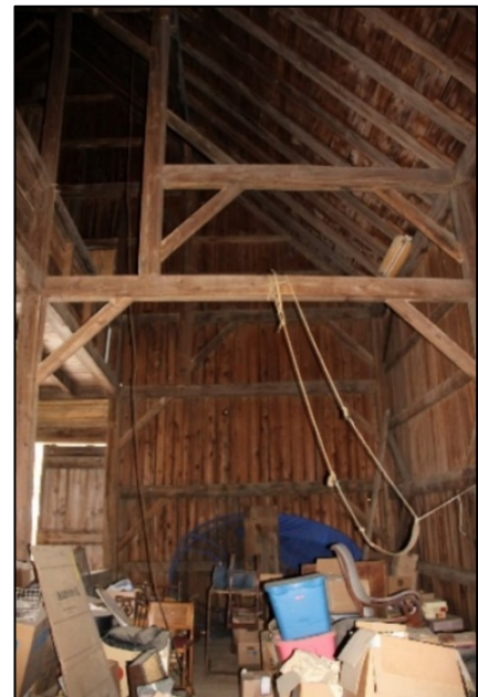
Bottom Right: Second floor hay loft and third floor bridge (on extreme left). This framing has the purlin supported on the tie beam. 2-story posts and a complex of tie beams support the bridge and roof
