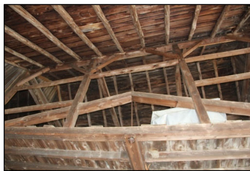
Bottom Left: Banked barn with high drive bridge at 1766 New Boston Road; Bottom Right: bridge truss structure of timbers and a metal rod, seen from below
